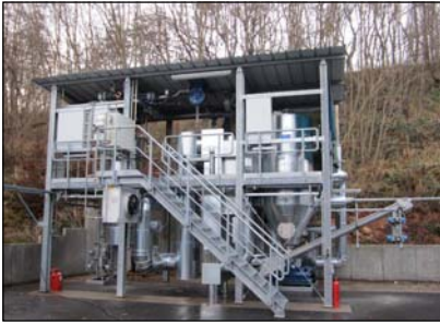
This IFF pilot plant recovers energy from fine grained residues
