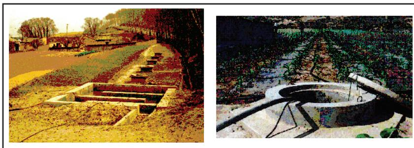
The sediment tank is used in case the catchment has a natural slope or some other earthen surface. The filtration facility is a small tank with gravel and sand placed layer by layer. The non-woven geomembrane wrapped outside an intake pipe of the tank can also be used as a filter.
